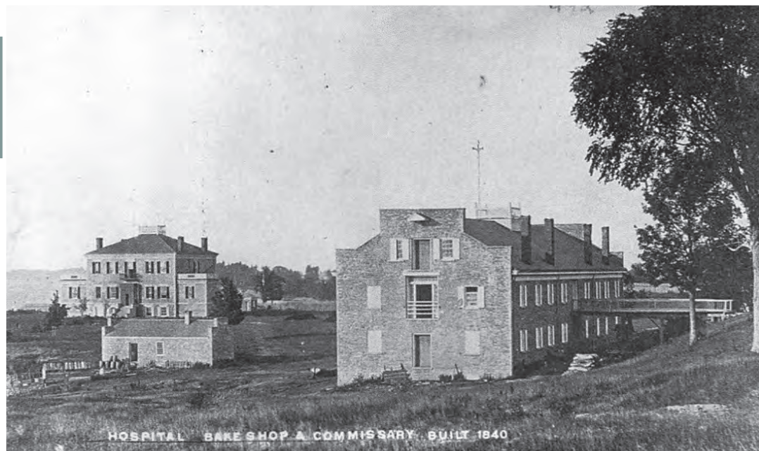
This photograph shows (from left) the post hospital, bakery, and commissary, all of which were constructed in 1839-40. (Sackets Harbor Historical Society)
